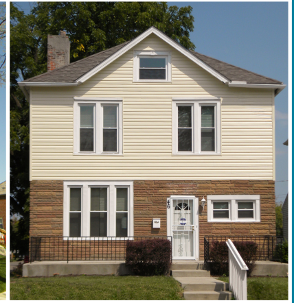
South Side Renaissance Homes
